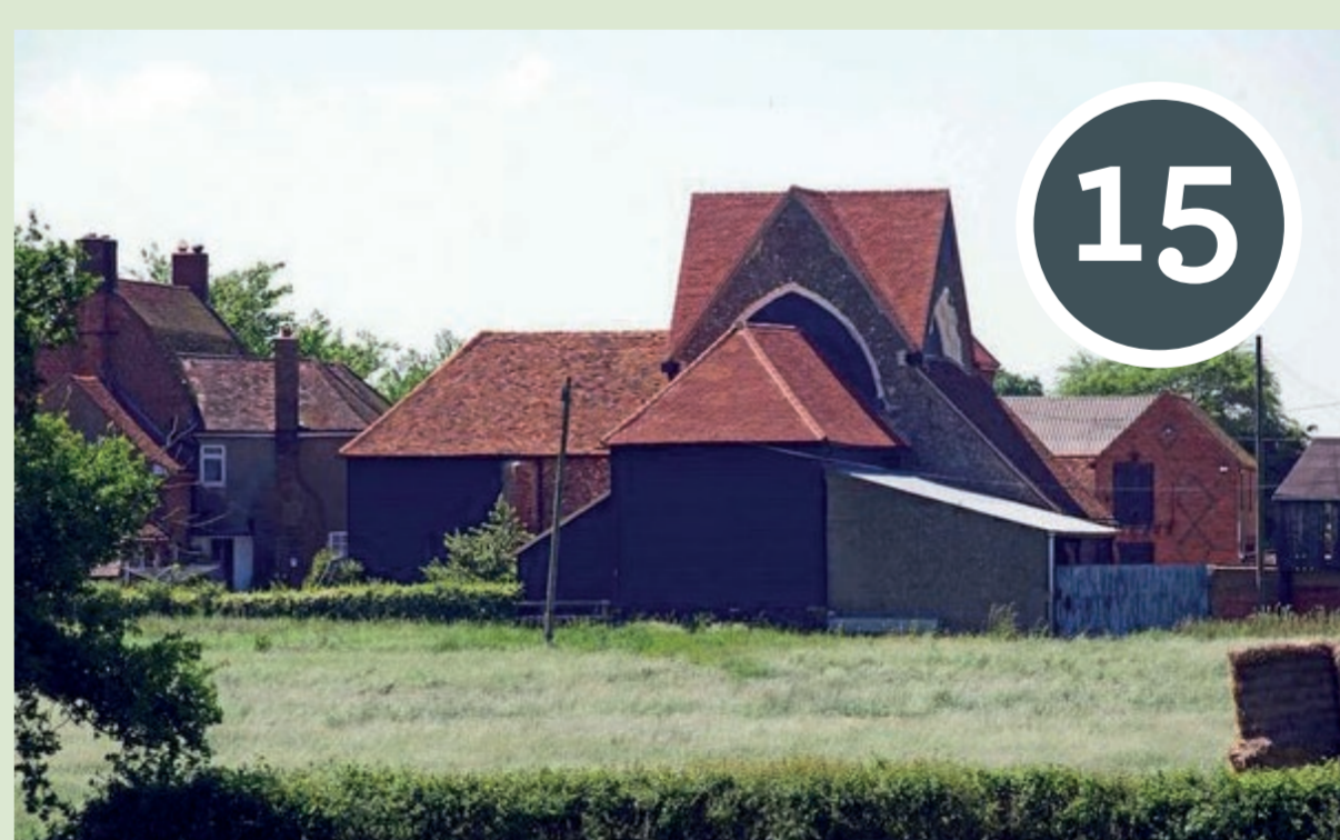
Latton Priory (Listed Building)
