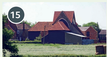
Latton Priory (Listed Building)
